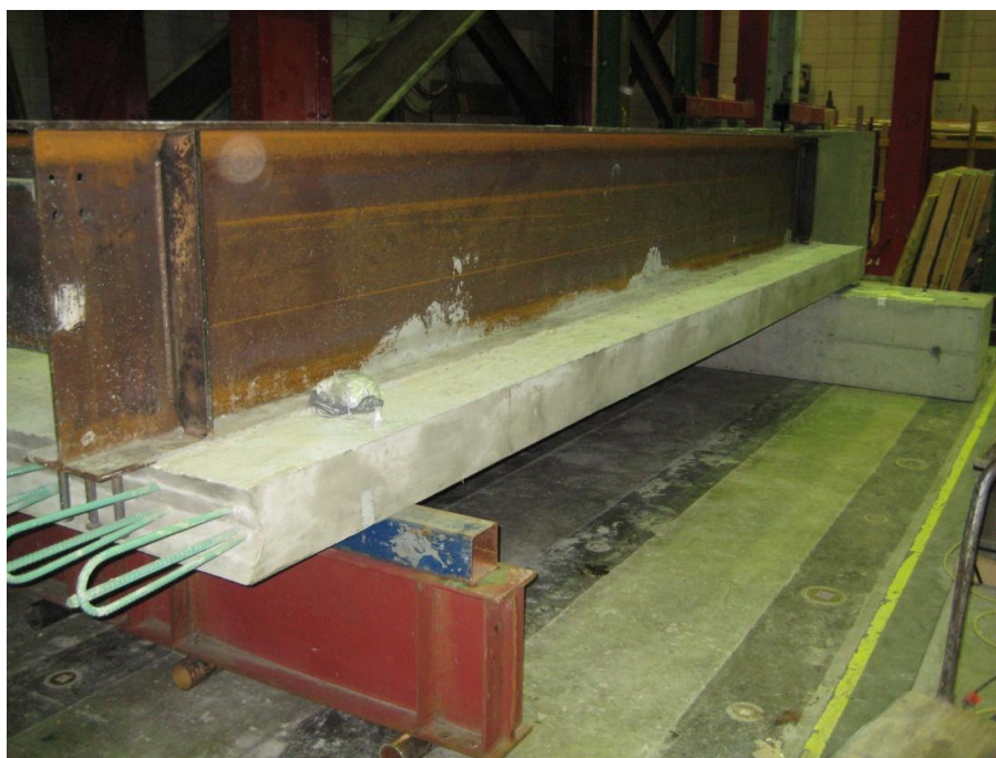
Figure 3.12. Completed Deck Module
