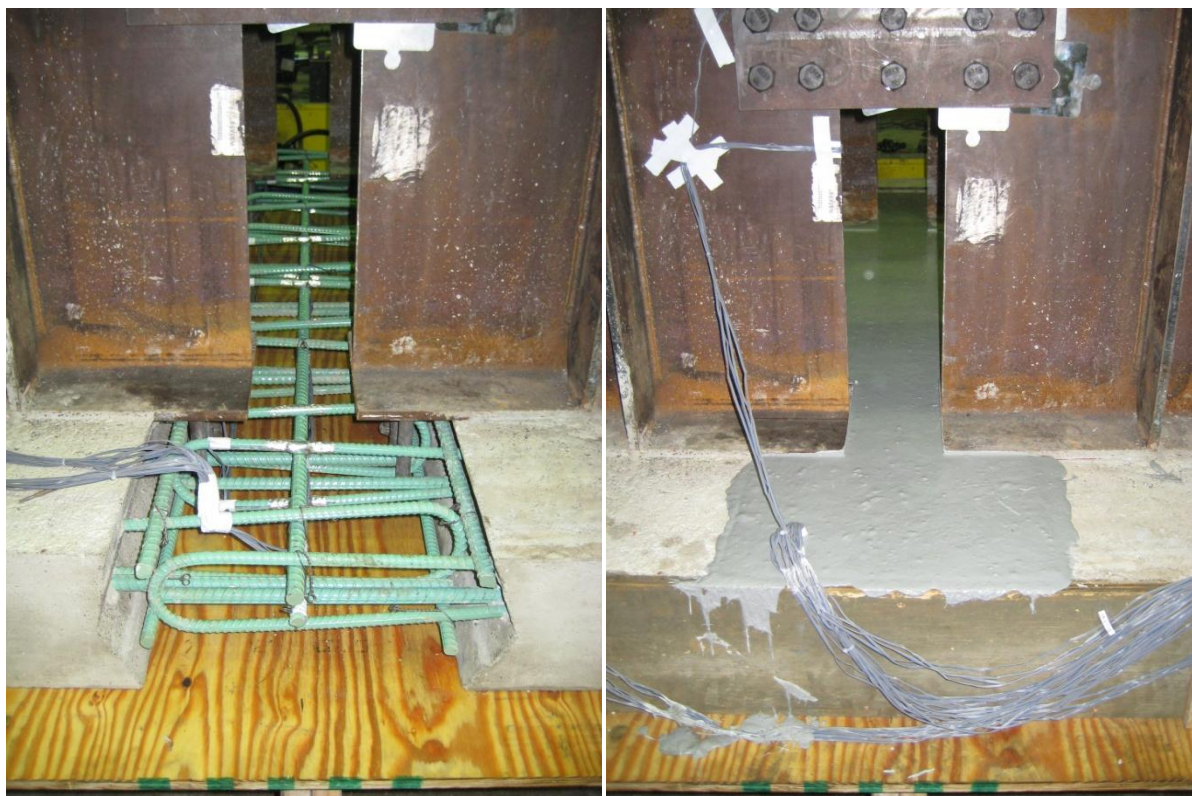
Figure 3.14. UHPC Joint Preparation and Placement
