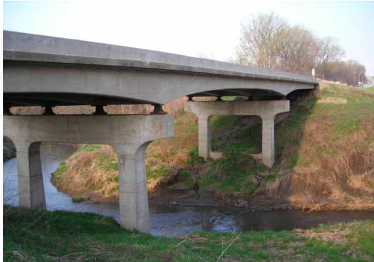
Figure 2.1. Existing US Highway 6 Bridge over Keg Creek
