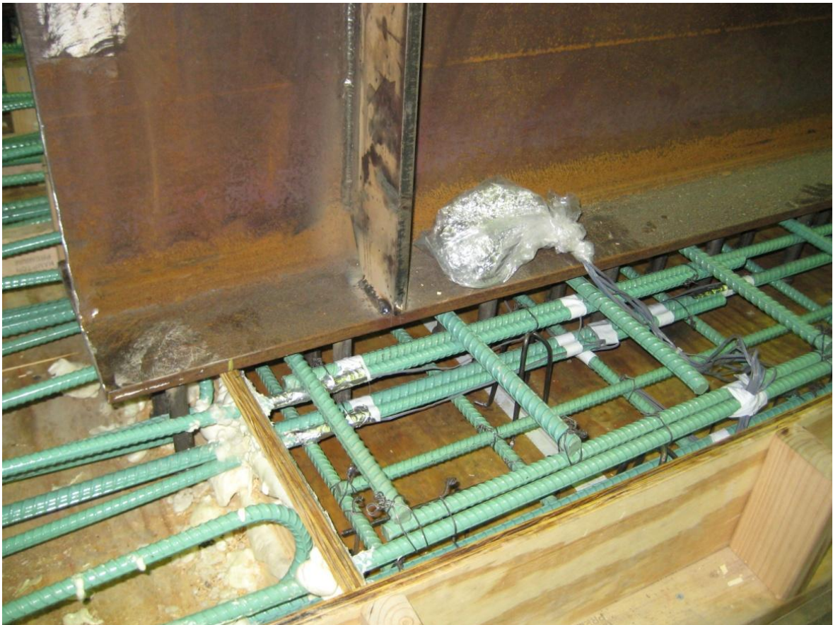
Figure 3.17. Embedded Bonded Strain Gages in HPC Deck
