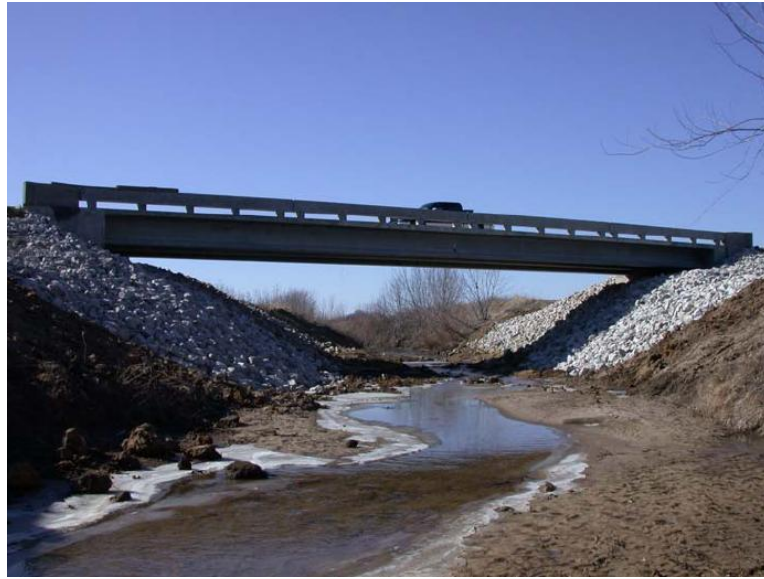
Figure 2.6. UHPC I-Girder Bridge - Wapello County, Iowa
