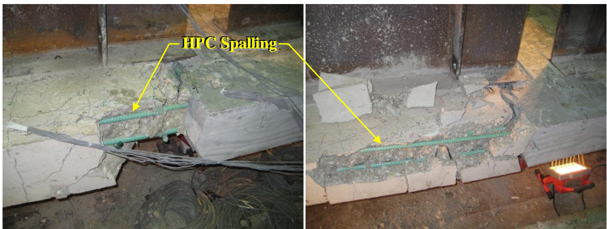
Figure 4.60. Exterior Hairpin Reinforcement (Opposite Sides)
