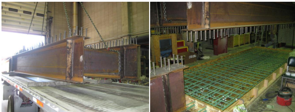
Figure 3.11. Prefabricated Deck Module Construction
