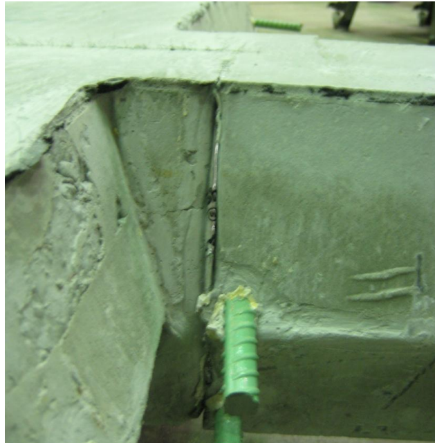
Figure 4.9. Stay-in-Place Acrylic Bulkhead
